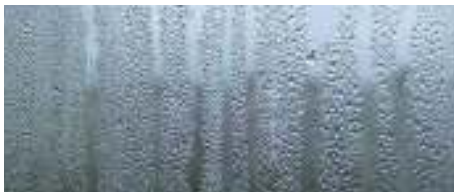
Condensation on the interior face of a DGU.
